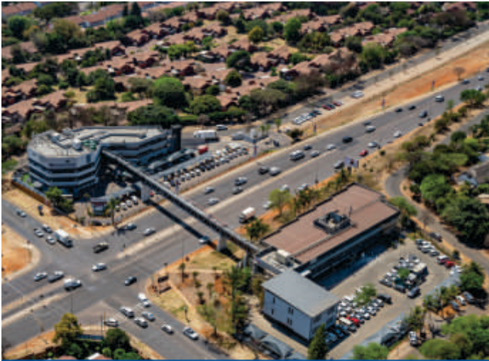
LIFE FAERIE GLEN REFURBISHMENT
