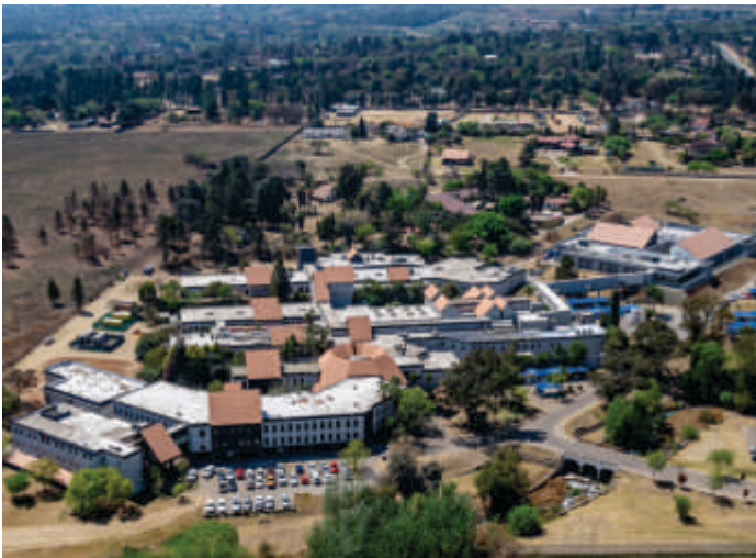
CARSTENHOF LIFE HOSPITAL REFURBISHMENT
